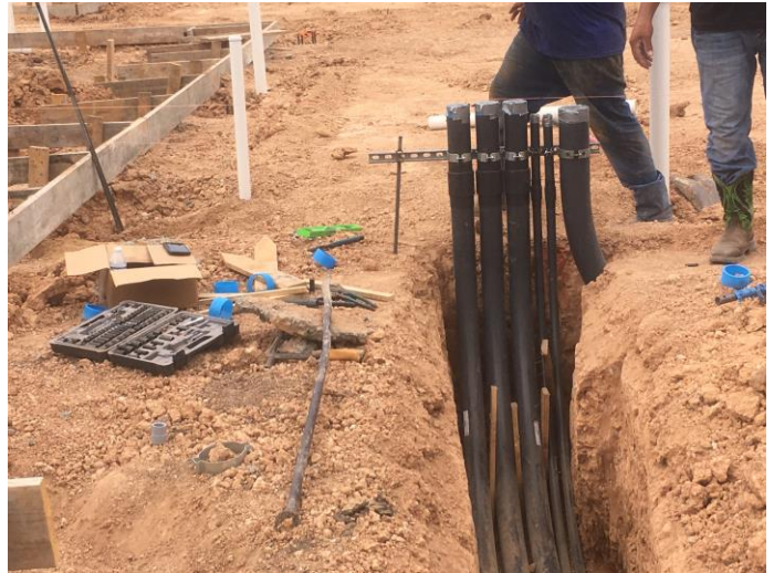
2. Underground electrical rough-in
