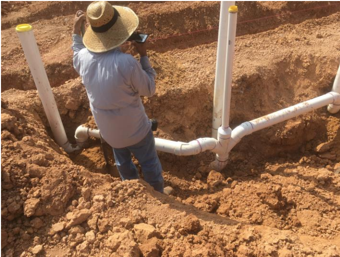
1. Underground plumbing rough-in
